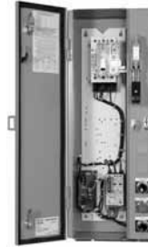
Type 12 Combination IT Starter with HMCPE
